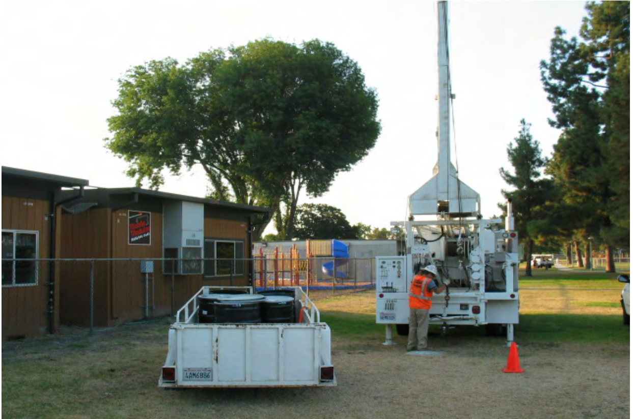
GMW-63 well development.
