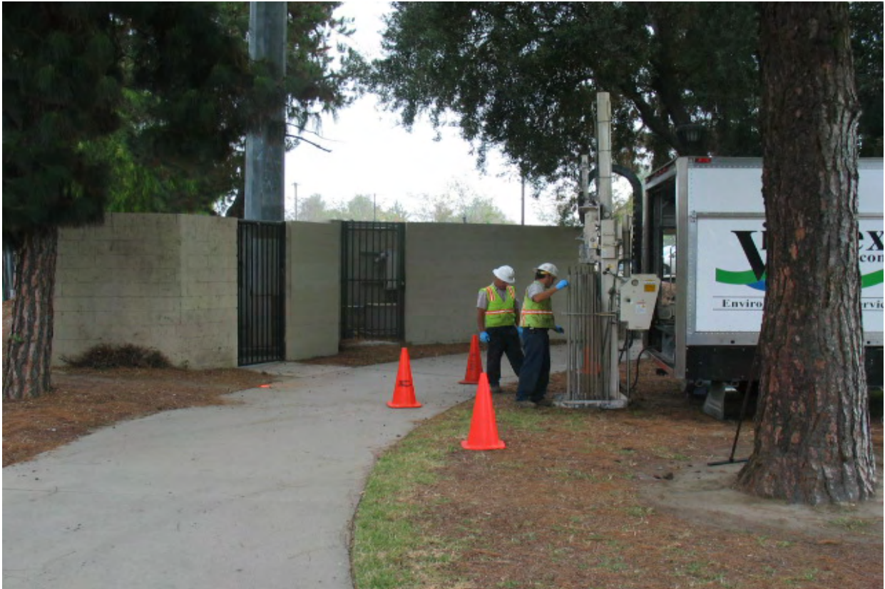
B-124 Hydropunch™ groundwater sampling.
