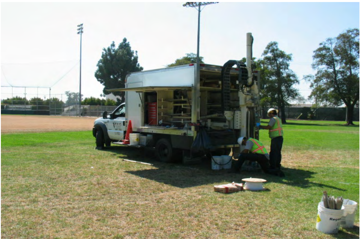
B-131 Hydropunch™ groundwater sampling.
