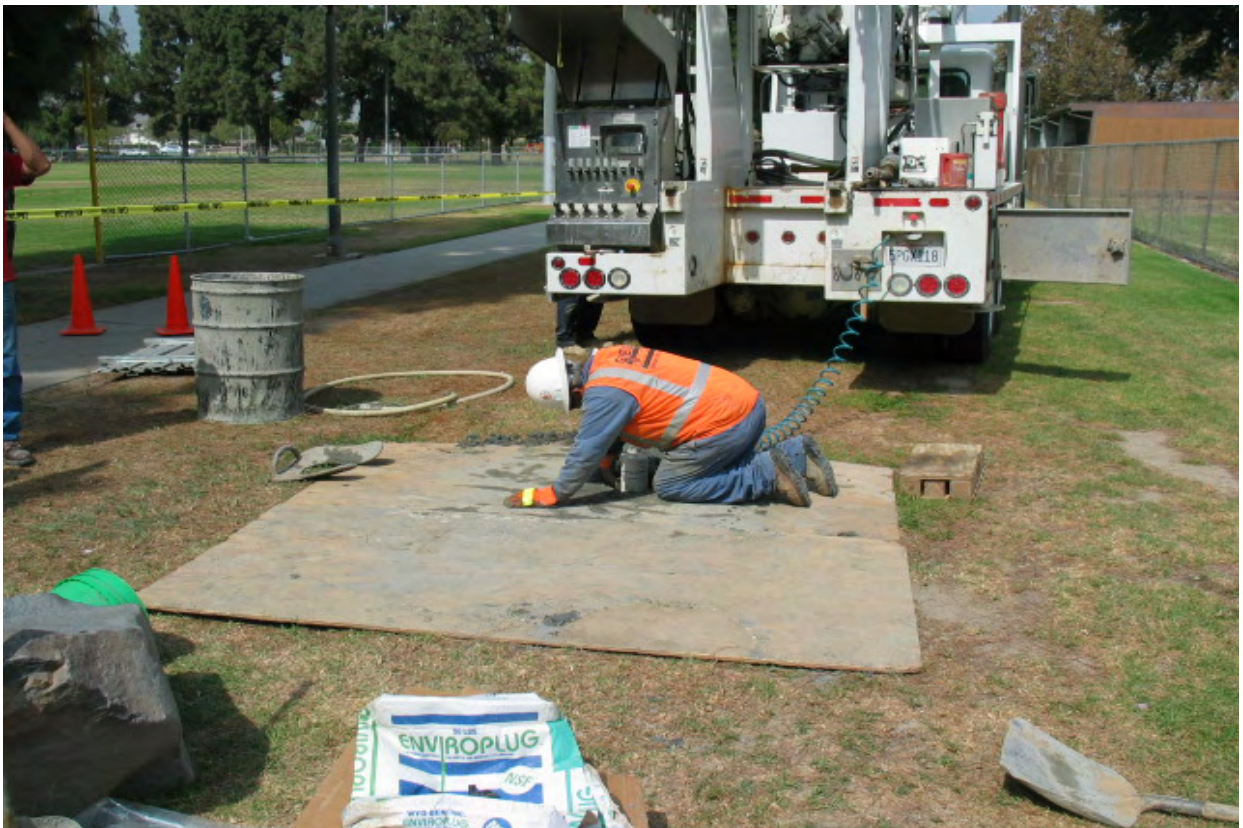
GMW-64 well installation.
