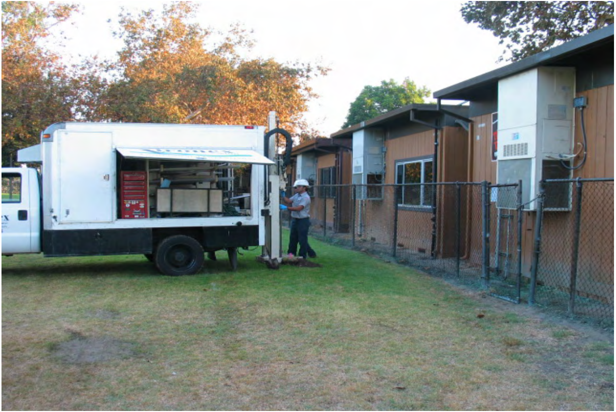
VMP-29 probe installation.
