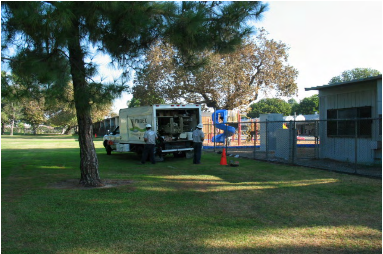
VMP-30 probe installation.
